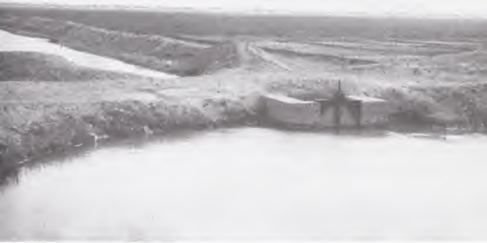
Control device for switching water flow to one of the many canals used for irrigation in Al Jazirah, south of Khartoum Courtesy Embassy of the Republic of Sudan, Washington
